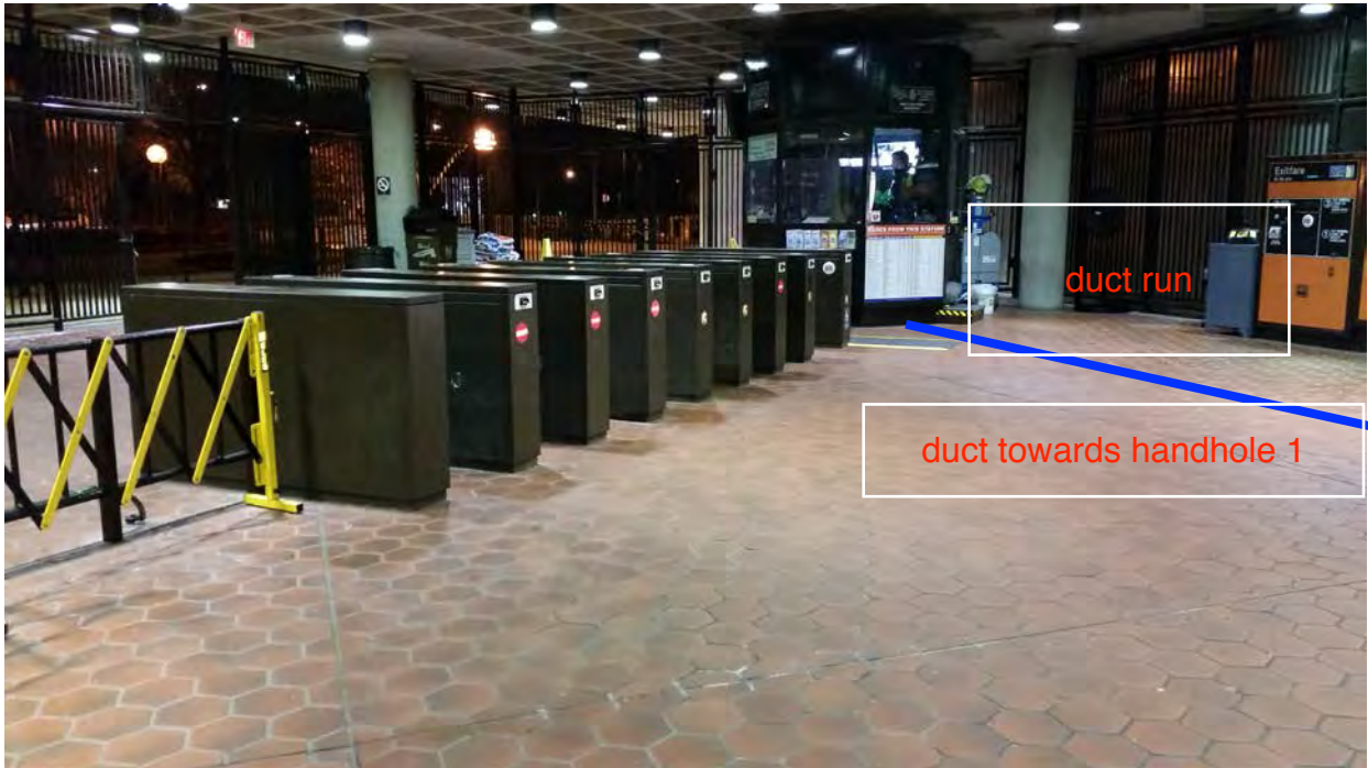
Photo #1 – E07 West Hyattsville: Duct run from kiosk towards handhole 1
